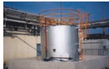
Unearthened fuel tank reinstalled above ground
